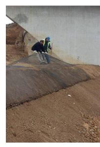
Top: The slope after installation, compaction and screeding off, but before the erosion control mat has been laid. Bottom: Laid using the fold-over method: rear-anchoring of the geogrid.
