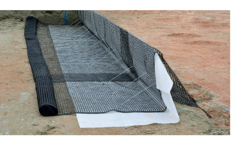
The structural steel angles are pre-bent in the factory according to the layer height and front inclination. An erosion control mat is attached to the inside of the structural steel angle for trickle protection. The geogrid is laid flat and then along the inside of the angle. The structural steel angle is also braced with steel bracing hooks. After the soil layer has been laid, the geogrid is folded back over the soil and integrated into the structure.
