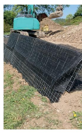
BEGREEN EASY can be used to create steep slopes with a front inclination of up to 70°. This system comprises a reinforcing geogrid, a bracing steel gabion mat and a hinged base grid as permanent formwork with bracing hooks and an erosion control mat. The system components are pre-assembled in the factory.
