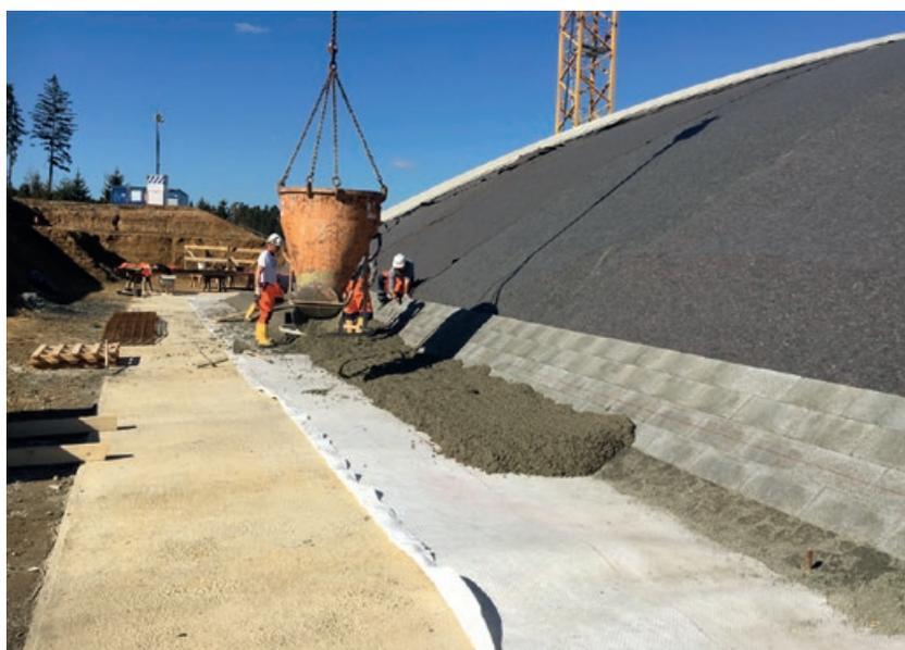
The use of a geosynthetic in place of conventional materials (with gravel fill material for drainage) has proven to be the more ecological solution.
