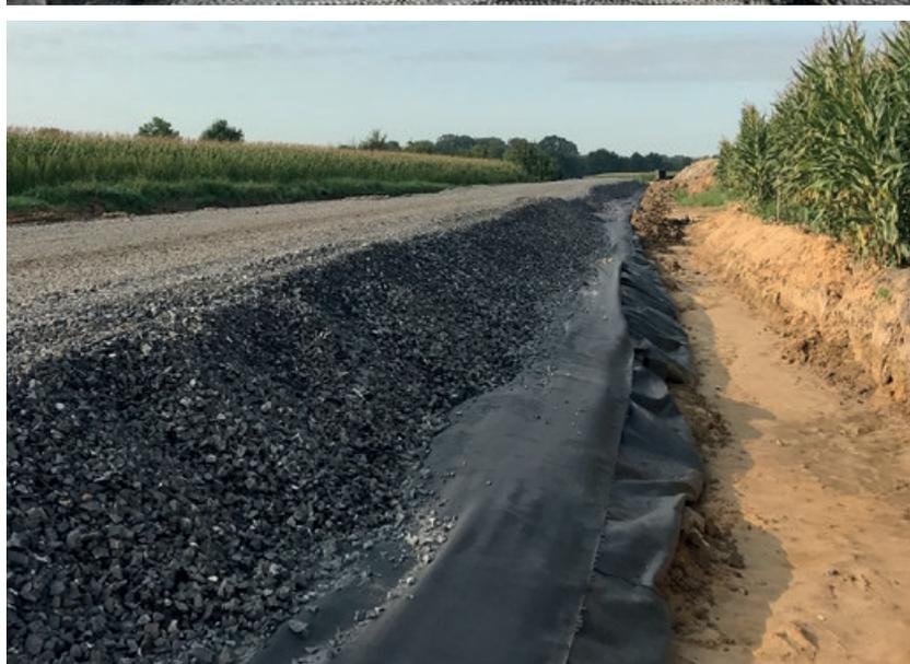
In the Drensteinfurt project, it was planned to use coarse fill material on a relatively deformable subsoil. The high loading applied during construction therefore required a material that surpassed even geotextile robustness class GRK 5.
