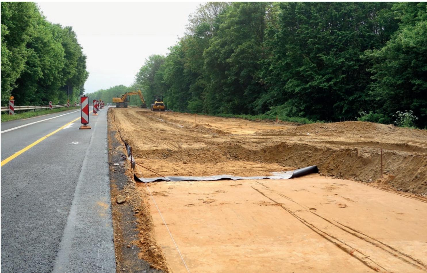
Reinforcing layer under roads with unbound surfaces (construction site access roads, service roads and access routes for site development)
