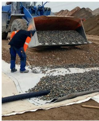
Construction of a sealed storage area for the temporary storage of concrete rubble and building rubble.
