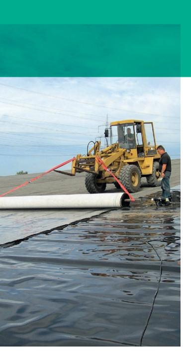
With mineral clay sealing layers, layer thicknesses of up to 100 cm are required. BENTOMAT achieves a comparable or superior sealing effect with a thickness of just 1 cm.
