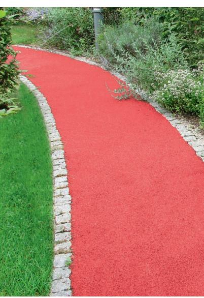
Two-layer construction for all areas requiring fall protection
