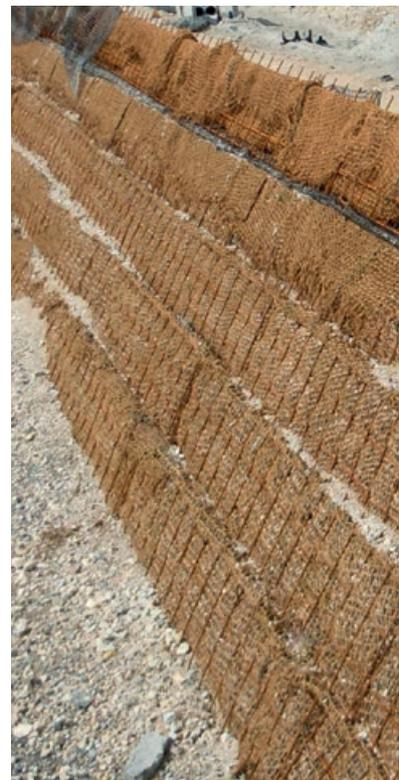
**BEGREEN 70 with welded and galvanised steel wire mesh mats**
