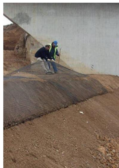
Top: The slope after installation, compaction and screeding off, but before the erosion control mat has been laid. Bottom: Laid using the fold-over method: rear-anchoring of the geogrid.
