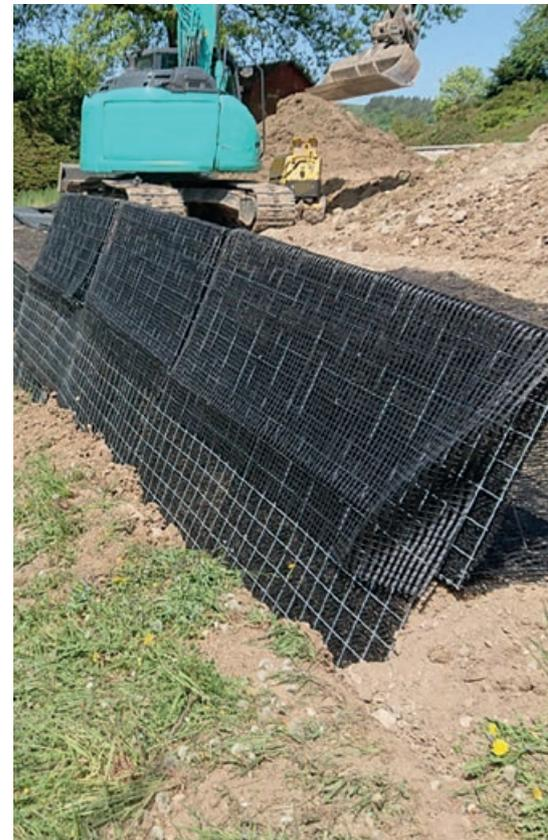
BEGREEN EASY can be used to create steep slopes with a front inclination of up to 70°. This system comprises a reinforcing geogrid, a bracing steel gabion mat and a hinged base grid as permanent formwork with bracing hooks and an erosion control mat. The system components are pre-assembled in the factory.
