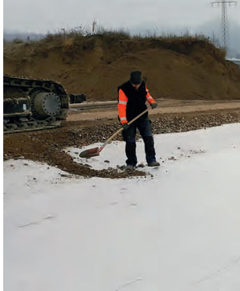
**BBO (Bodenseekreis Bauschutttaufbereitung GmbH & Co. KG) operates a collection point on the premises of the Hardt GmbH & Co. KG gravel plant. The mineral rubble that is stored here temporarily is used to produce recycled construction materials. The storage and operating area needed to be constructed in such a way that surface water could be discharged and soaked away in a controlled manner. The original design envisaged the construction of a waterproof concrete slab.**
