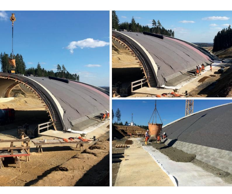
The use of a geosynthetic in place of conventional materials (with gravel fill material for drainage) has proven to be the more ecological solution.
