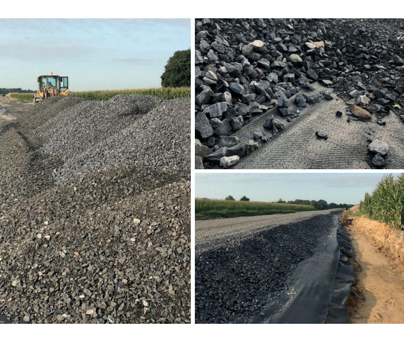
In the Drensteinfurt project, it was planned to use coarse fill material on a relatively deformable subsoil. The high loading applied during construction therefore required a material that surpassed even geotextile robustness class GRK 5.
