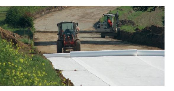
Separation and filtration are the primary functions performed by BONTEC NW Non-woven Fabrics in earthworks and traffic infrastructure.
