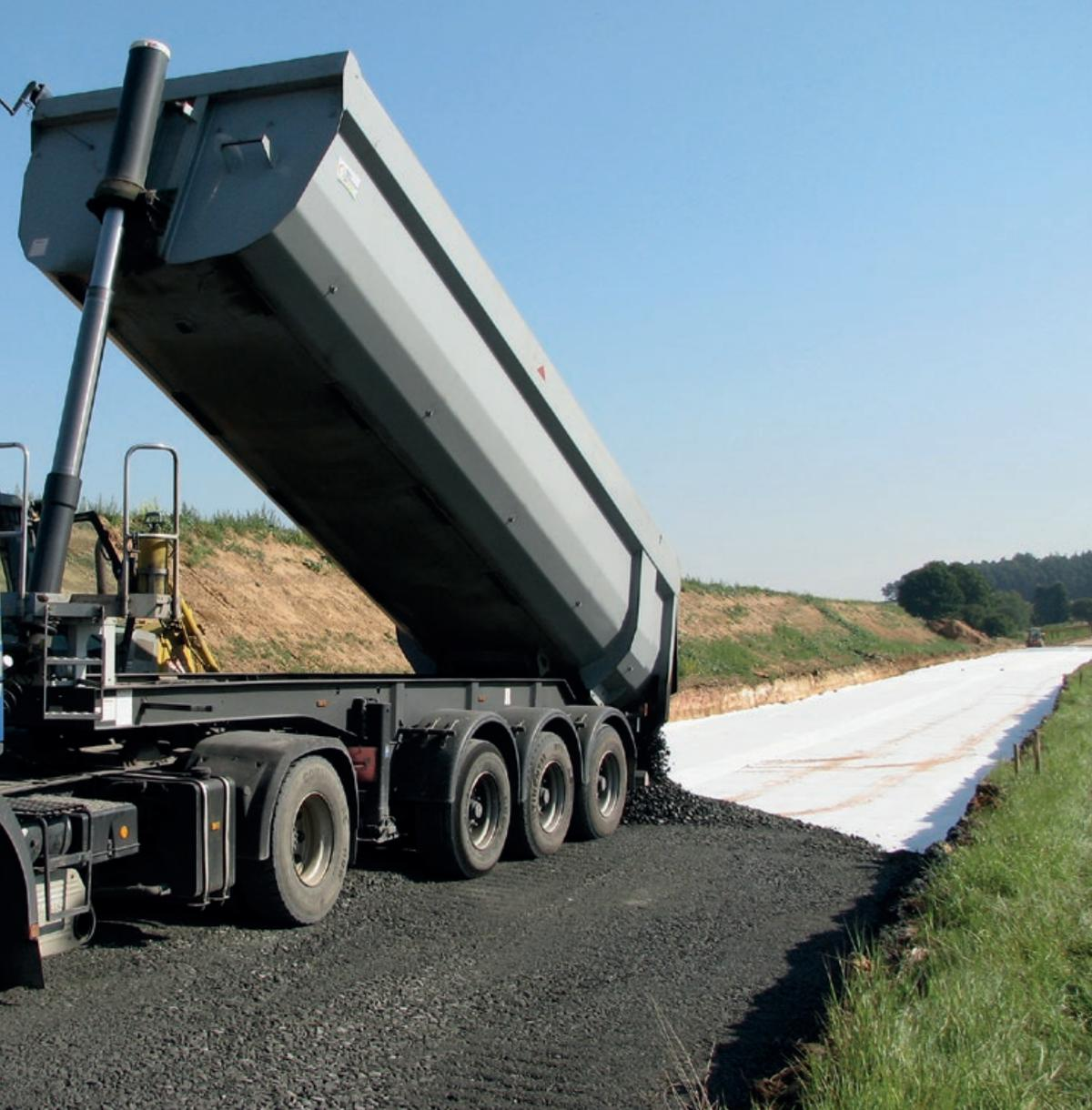
Important parameters for the allocation to GRK classes include the soil class and grain shape of the soil to be filtered, the load applied by the fill material, and also the stresses encountered during the installation and construction works. The type and method of installation and compaction of the fill material are just as relevant as the expected loading by construction traffic.
